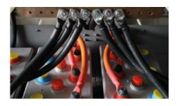
a large off grid system that consisted of a 6080Ah battery bank and 9 x Quattro 48/10000/140.
