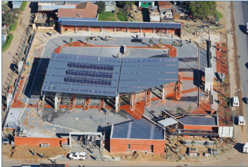
“One of the most exciting features of this facility is the manner in which we are using the rank’s considerable roof area for the harvesting of rainwater. The rainwater is stored in an underground tank system with a storage capacity of up to 20 000 litres and is equipped with the necessary infrastructure to pump this water to the washing bays,” said Councillor Herron.
