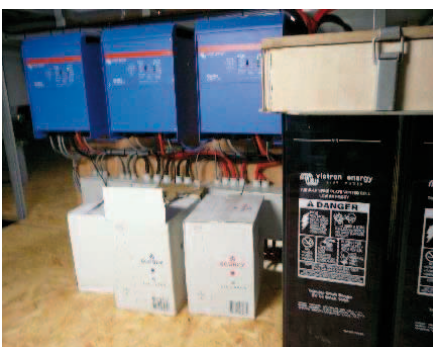
Battery bank 1500Ah-24Vdc
