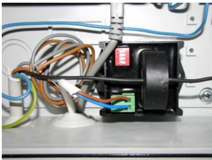
In the above image an installation cable 2 × 0.75mm<sup>2</sup> is used for connecting the sensor to the ECOMulti. Tests have shown, that a shielded cable doesn't improve the values. An installation cable is enough. The brown wire is plus, the blue wire is minus!
