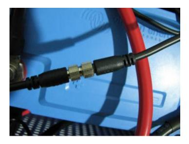
Connect the BMS cables to the VE.Bus BMS in the ECOmulti:
