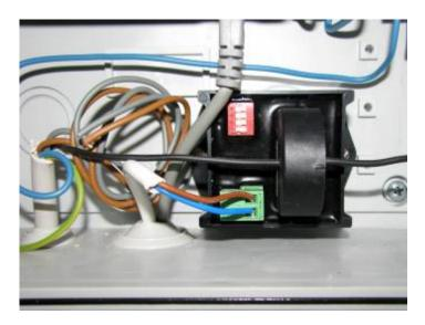
In the above image an installation cable  $2 \times 0.75 \text{mm}^2$  is used for connecting the sensor to the ECOmulti. Tests have shown, that a shielded cable doesn't improve the values. An installation cable is enough. The brown wire is plus, the blue wire is minus!
