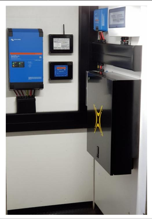
== Typical installation with Multiple SS202 modules, 3 Quattros, 3 MPPTs, and Fronius integration ==
