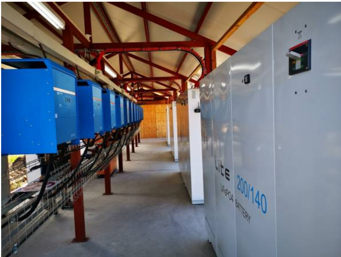
Figure 2 Typical Installation: 7 x Freedom Lite Commercial 200/140 with Victron 12 x 15kVA Quattro and 10 x Ve Direct MPPT's and 6 x Fronius ECO 27kW
