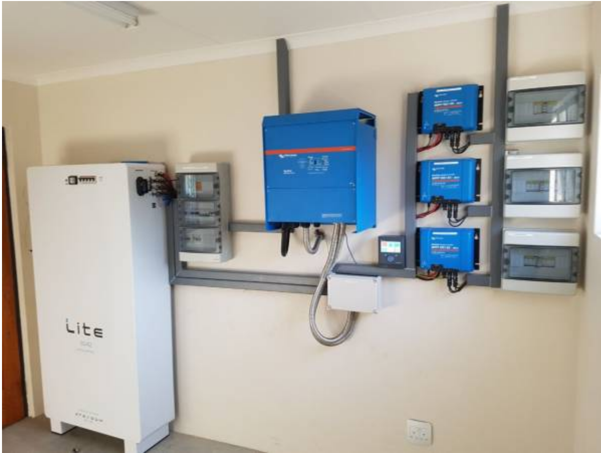
Figure 2 Typical Installation: 7 x Freedom Lite Commercial 200/140 with Victron 12 x 15kVA Quattro and 10 x Ve Direct MPPT's and 6 x Fronius ECO 27kW
