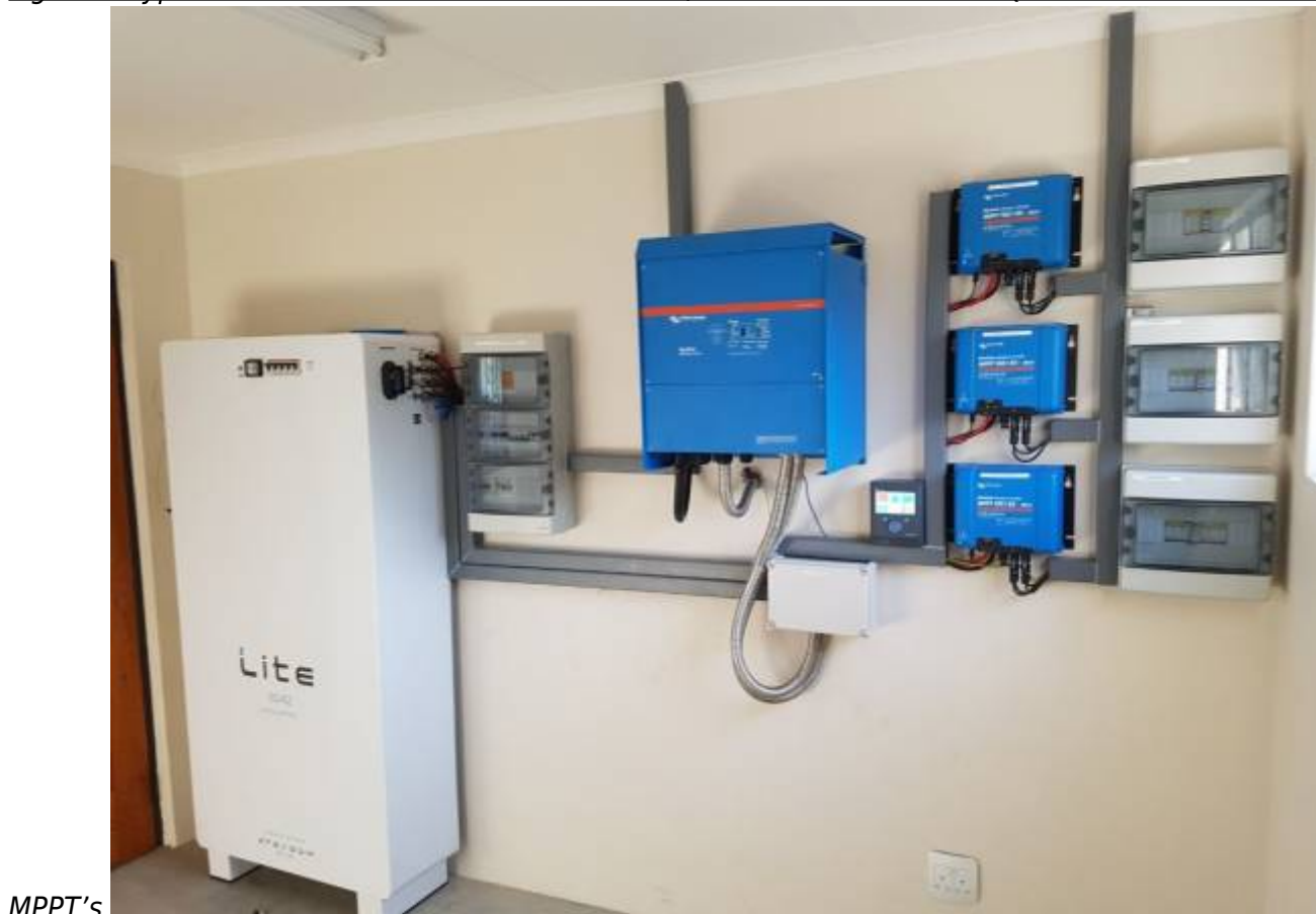
Figure 1 Typical Installation: Freedom Won LiTE 60/42 with Victron 15kVA Quattro and 3x Ve Direct
