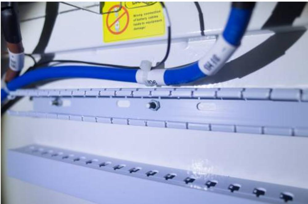
This seems really bad design as there is the possibility that the metal screws could damage the single insulated battery cables.
