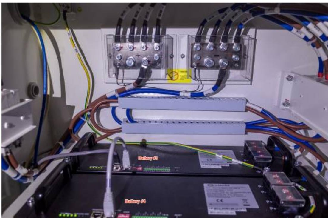
The top end of the cable went into the left port of battery#3. Finally the COMout of the third jumper went into the right port of battery #3 and the COMin went into the right port of battery #4.
